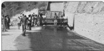
Sealing works by double Ottaseal.
