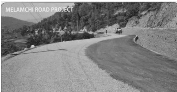
Sealing works by double Ottaseal.
